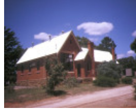
1 guildford primary school number 264 franklin street guildford corner view jan1989
