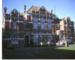
1 ballarat high school sturt street west ballarat front view apr1987
