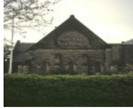
1 christ church complex church square st kilda west front of church
