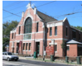
ALL SAINTS CHURCH, HALL AND FORMER VICARAGE SOHE 2008
