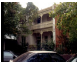
St Marks George St Fitzroy Vicarage
