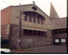
St Marks George St Fitzroy Former Sunday School
