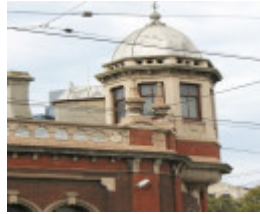
FORMER CABLE TRAM ENGINE HOUSE SOHE 2008
