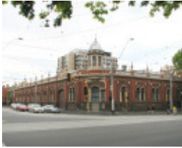
FORMER CABLE TRAM ENGINE HOUSE SOHE 2008
