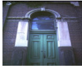
cable tram engine house gertrude street fitzroy detail front entrance
