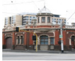
FORMER CABLE TRAM ENGINE HOUSE SOHE 2008
