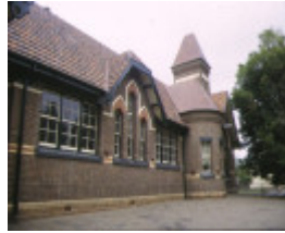
1 primary school 773 caulfield south window detail
