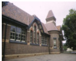
1 primary school 773 caulfield south window detail
