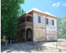
GREGORYS BRIDGE HOTEL SOHE 2008
