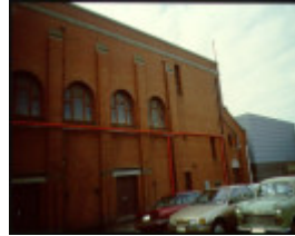
H01967 cathedral hall south elevation
