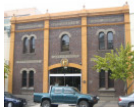
Former Veterinary Hospital Fitzroy 26 March 2008 mz Front Elevation
