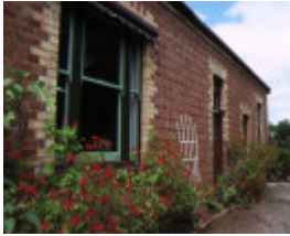
millbank grant street bacchus marsh side view windows and brickwork
