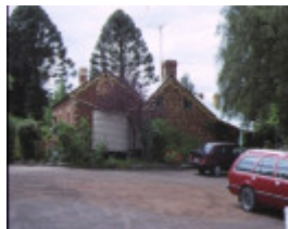
1 millbank grant street bacchus marsh rear view of homestead
