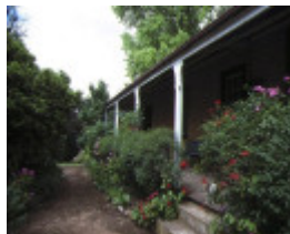
millbank grant street bacchus marsh verandah
