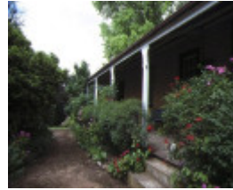
millbank grant street bacchus marsh verandah
