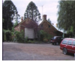
1 millbank grant street bacchus marsh rear view of homestead
