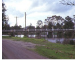
1 bridge broken river benalla side view 1989
