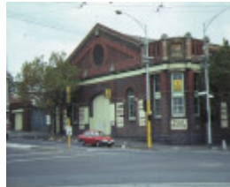
former cable tramway engine house abbotsford street north melbourne front view
