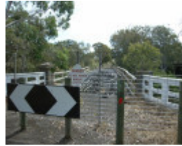
ELLERSLIE BRIDGE SOHE 2008
