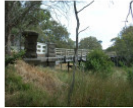
ELLERSLIE BRIDGE SOHE 2008
