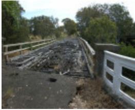
ELLERSLIE BRIDGE SOHE 2008
