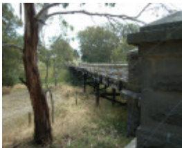
ELLERSLIE BRIDGE SOHE 2008
