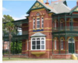
BUNDOORA PARK HOMESTEAD SOHE 2008
