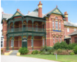
BUNDOORA PARK HOMESTEAD SOHE 2008
