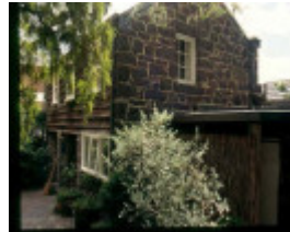
H00162 35 hanover street former stables
