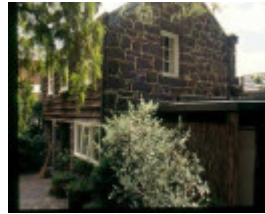
H00162 35 hanover street former stables
