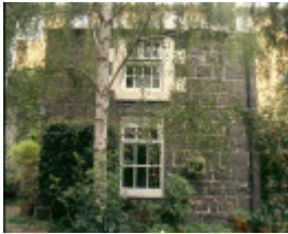
H00162 35 hanover street fitzroy kitchen block
