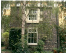
H00162 35 hanover street fitzroy kitchen block
