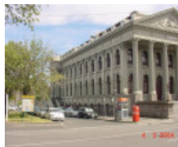
h00147 fitzroy town hall napier street fitzroy side she project 2004
