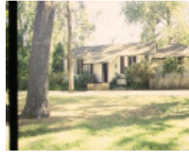
1 la trobe cottage 162 birdwood avenue south yarra front view
