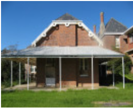
Bairnsdale Hospital rear of north wing
