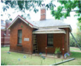
FORMER LANDS OFFICE SOHE 2008
