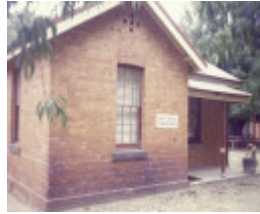
h01069 former lands office arundel street benalla front she project 2004
