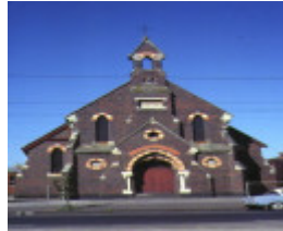
1 methodist church nicholson street fitzroy front elevation apr1978
