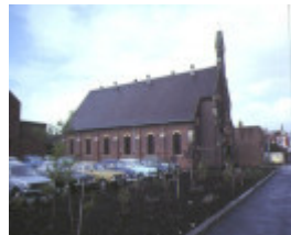
methodist church nicholson street fitzroy side elevation aug1980
