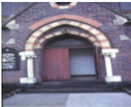
methodist church nicholson street fitzroy entrance aug1980
