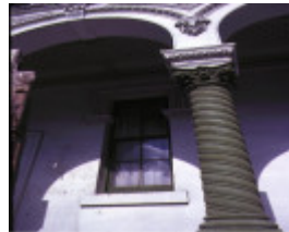
residence 122 nicholson street fitzroy balcony column detail
