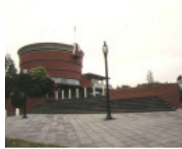
1 brighton municipal offices side view
