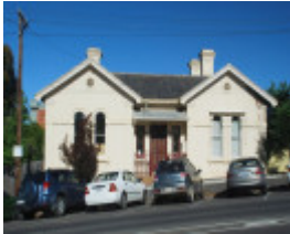
FORMER GOLD WARDEN'S OFFICE SOHE 2008
