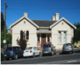
FORMER GOLD WARDEN'S OFFICE SOHE 2008
