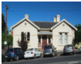
FORMER GOLD WARDEN'S OFFICE SOHE 2008
