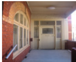
Prahran Volunteer Fire Station_Front Porch_Jan 2008_mz
