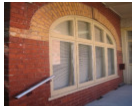
Prahran Volunteer Fire Station_Former Front Door_Jan 2008_mz
