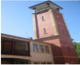
Prahran Volunteer Fire Station_Watchtower_Jan 2008_mz
