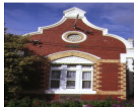
1 coppin avenue 8 coppin avenue front window aug1990
