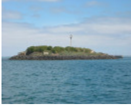
SOUTH CHANNEL FORT SOHE 2008
