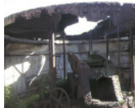
1 south channel fort gun emplacement jun1989
