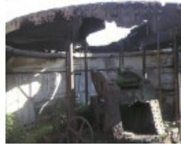
1 south channel fort gun emplacement jun1989
