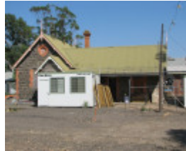
PRIMARY SCHOOL NO. 1975 SOHE 2008
