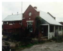
H01098 rafa barracks horse hospital demolished 1995
