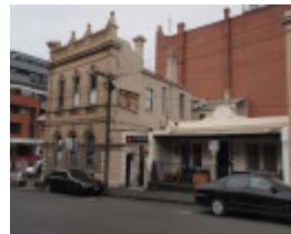
H0506 FORMER UNION BANK OF AUSTRALIA LHA 2015 3.JPG
