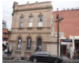
H0506 FORMER UNION BANK OF AUSTRALIA LHA 2015 2.JPG
