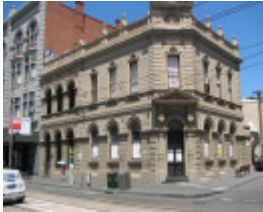
FORMER UNION BANK OF AUSTRALIA SOHE 2008
