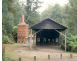
H02012 kurth kiln and storage shed
