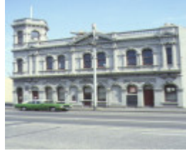
former north fitzroy port office st georges road fitzroy front elevation
