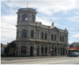
FORMER NORTH FITZROY POST OFFICE SOHE 2008
