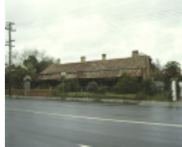
1 iron cottage brunswick road brunswick housing row 1992
