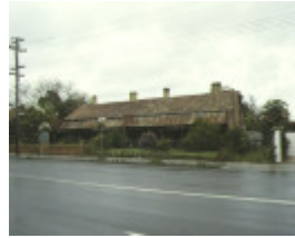
1 iron cottage brunswick road brunswick housing row 1992
