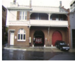
1 hawthorn fire station front view
