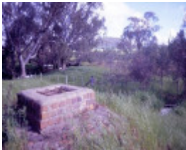
h01330 former thooona dairy and butter factory sargeant street thooona over underground water tank she project 2004
