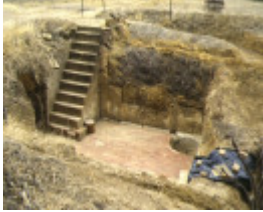
1 former thooona dairy & butter factory foundations
