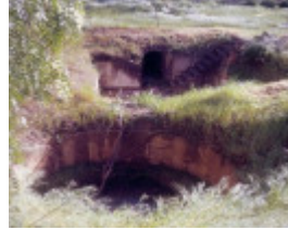
h01330 former thooona dairy and butter factory sargeant street thooona over butter factory remains she project 2004
