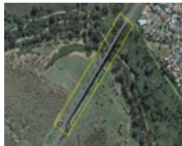
Albion Viaduct Extent Aerial June 2021
