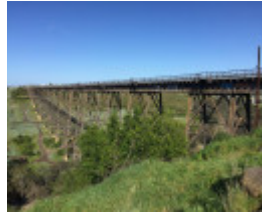
RAIL BRIDGE (ALBION VIADUCT) September 2016
