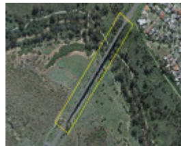
Albion Viaduct Extent Aerial June 2021
