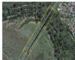
Albion Viaduct Extent Aerial June 2021
