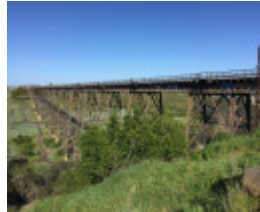
RAIL BRIDGE (ALBION VIADUCT) September 2016
