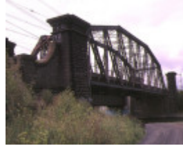
1 rail bridge over maribyrnong river footscray end view apr1996
