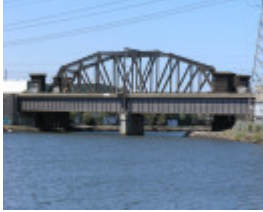
RAIL BRIDGE SOHE 2008
