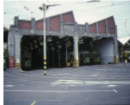
1 essendon tramway depot mount alexander road ascot vale saw tooth roof of tran shed
