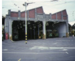
1 essendon tramway depot mount alexander road ascot vale saw tooth roof of tran shed
