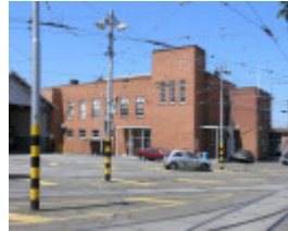
ESSENDON TRAMWAY DEPOT SOHE 2008
