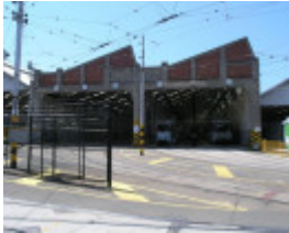
ESSENDON TRAMWAY DEPOT SOHE 2008
