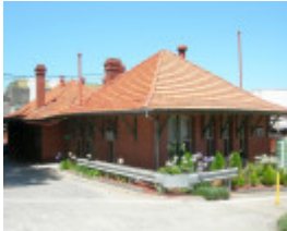
JENNERIAN BUILDING SOHE 2008
