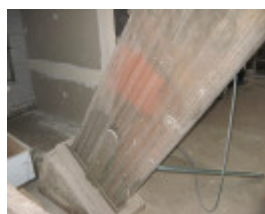
glue laminated beam abutment
