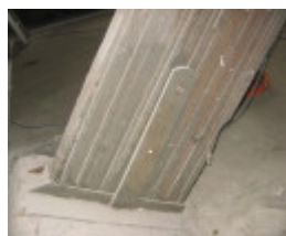
glue laminated beam abutment
