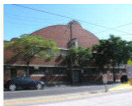
FORMER BURGE BROS FACTORY SOHE 2008
