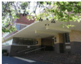
FORMER ESSENDON TECHNICAL SCHOOL SOHE 2008
