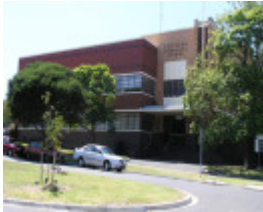
FORMER ESSENDON TECHNICAL SCHOOL SOHE 2008
