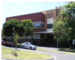
FORMER ESSENDON TECHNICAL SCHOOL SOHE 2008
