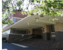
FORMER ESSENDON TECHNICAL SCHOOL SOHE 2008
