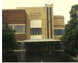
1 former essendon technical school buckley street essendon front entrance
