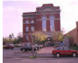
former north fitzroy electric railway substation brunswick street north fitzroy front view jun1995
