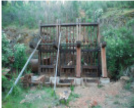
WALLABY MINE GOLD BATTERY SITE SOHE 2008
