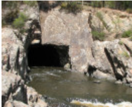
POUND BEND GOLD DIVERSION TUNNEL SOHE 2008
