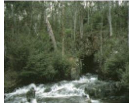
1 delegate river gold diversion tunnel bonang entrance view
