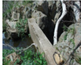
HOUGHTONS FLAT GOLD DIVERSION TUNNEL SOHE 2008
