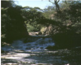
1 harrison's cut diversion sluice dargo river dargo front view
