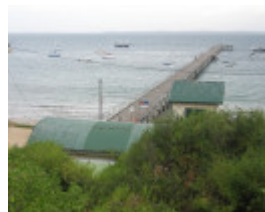
Jetty & shed - view from hill, Jan 2008
