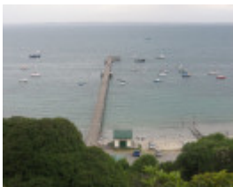
Jetty & surrounds - view from hill, Jan 2008
