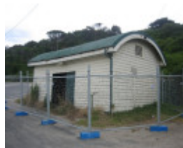
Former jetty cargo shed - view from north east, Jan 2008
