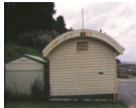
former jetty cargo shed flinders foreshore flinders rear shed side view
