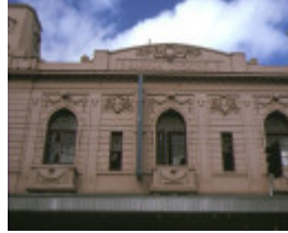
former barkley theatre barkly street footscray front windows aug1990
